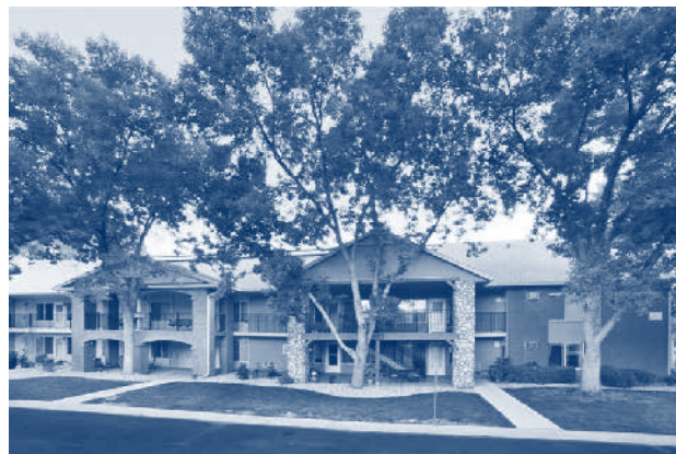
Photo Credit: Courtesy of FirstBank, Funding Partners, and Fort Collins Housing Authority
